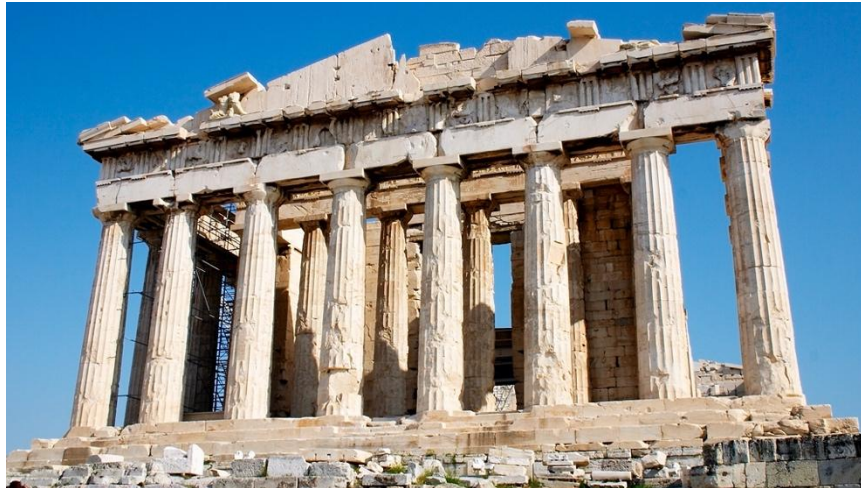
Figure 12. An example of colonnade, a row of columns that support a roof, as demonstrated in this picture of the Parthenon. Their purpose is both structural and aesthetic. From Image Parthenon-Restoration-Nov-2005-a, by Barcex, 2005 https://commons.wikimedia.org/wiki/File%3AParthenon-Restoration-Nov-2005-a.jpg . © 2005 by Barcex
